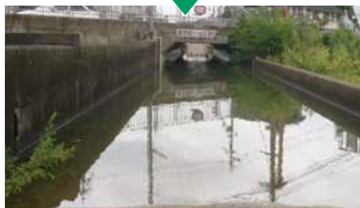
Underpass in a flood
