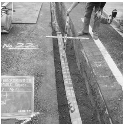
老朽管の敷設替え
